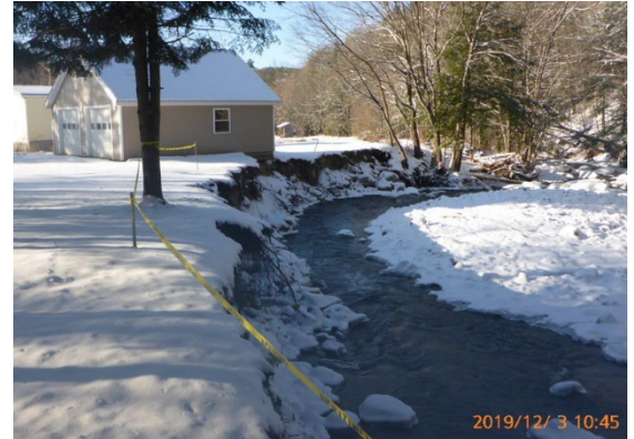
Due to extreme rainfall on October 31, 2019, Lewis Creek in the Town of Bristol, Vermont, had extensive flood flows which caused bank erosion that endangered a two garage and residence.
