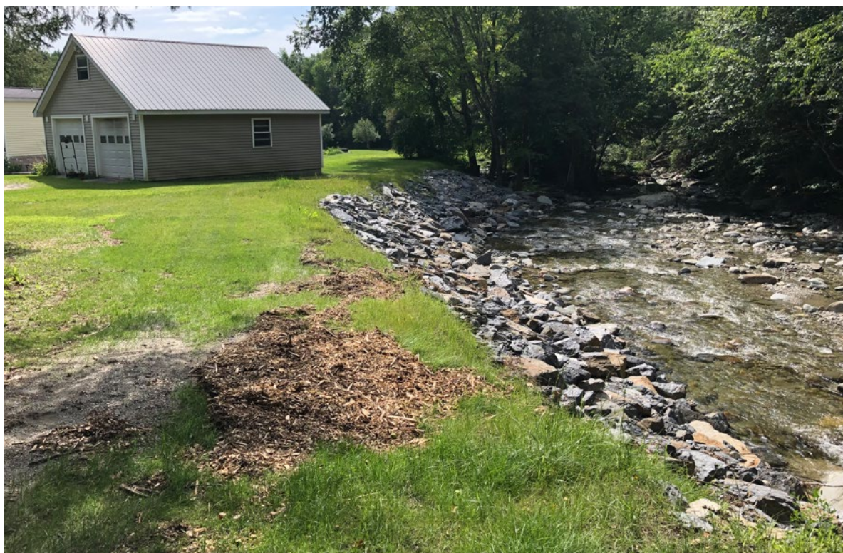
After EWP repairs, the streambank has been stabilized to prevent further bank erosion and danger to the buildings.
