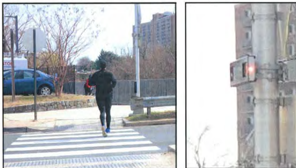
Figure 2. View of pilot light to pedestrian at shared-use path crossing with median refuge. Enlargement of pilot light at right.
