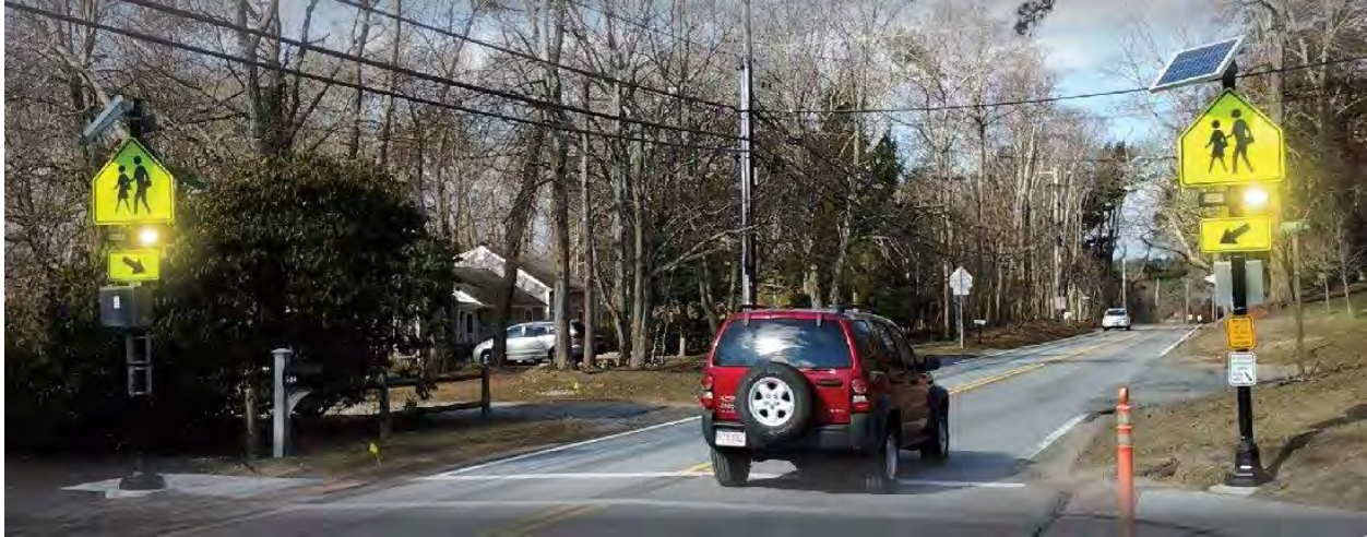
Figure 1 - Gate-posted RRFB installation at a school crosswalk
