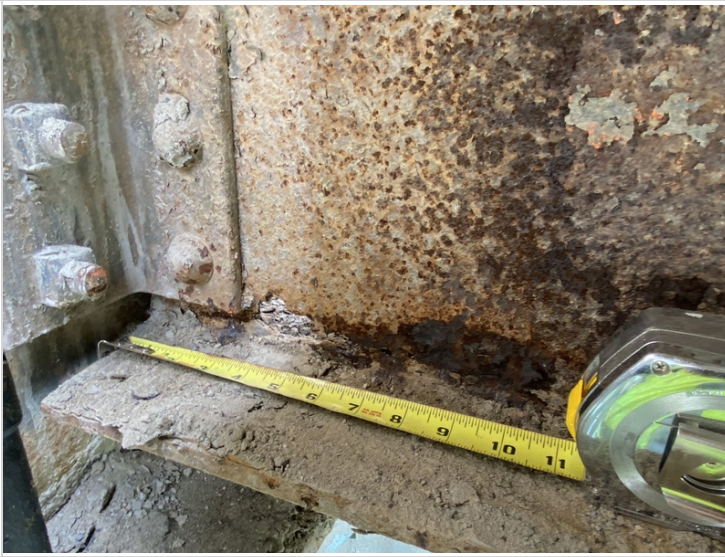
Floorbeam #1 on Downstream Side
