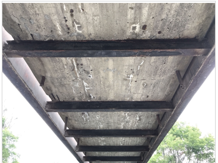
Soffit & superstructure facing abutment 1
