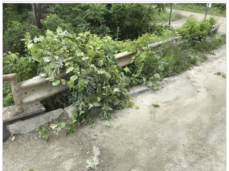
Upstream approach rail to abutment 2
