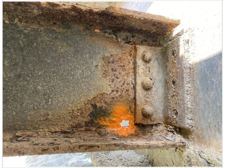
Floorbeam #3 on Downstream Side
