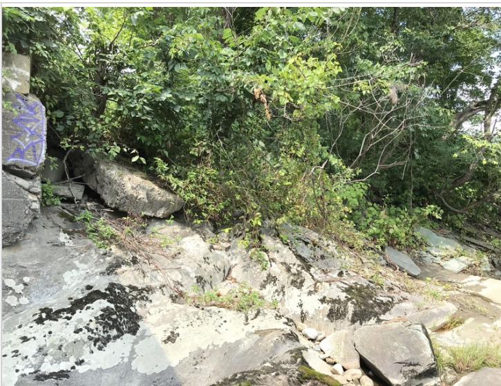
Downstream of abutment 2
