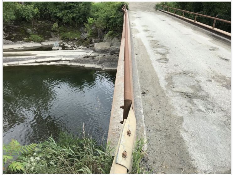
Upstream beam & rail from abutment 1
