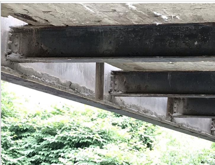
Downstream ends of floor beams 4 thru 6
