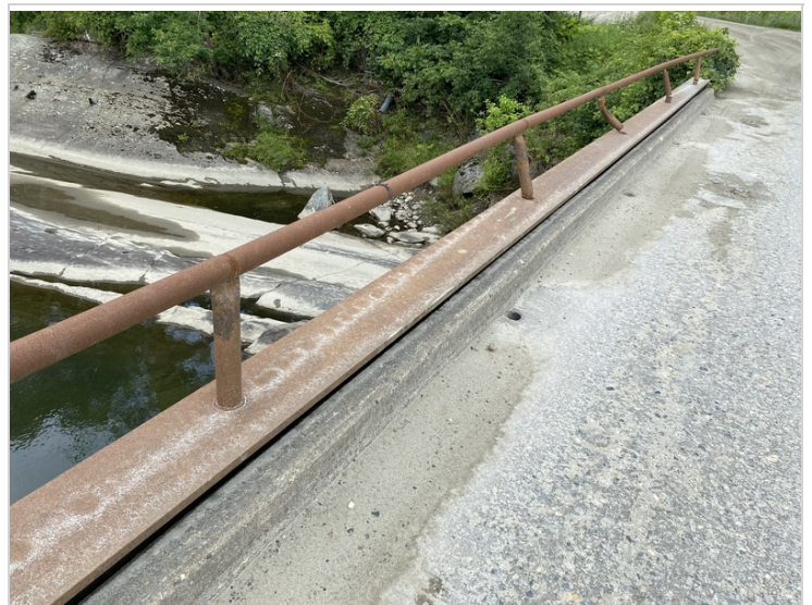
Upstream Bridge Rail Post #5 to Post #10
