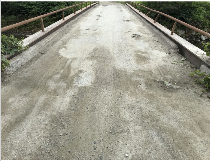
Wearing surface from abutment 2
