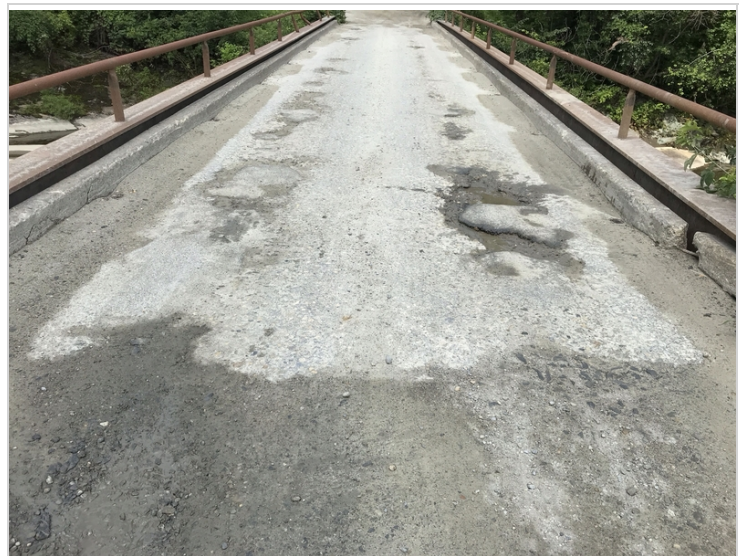
Wearing surface from abutment 1
