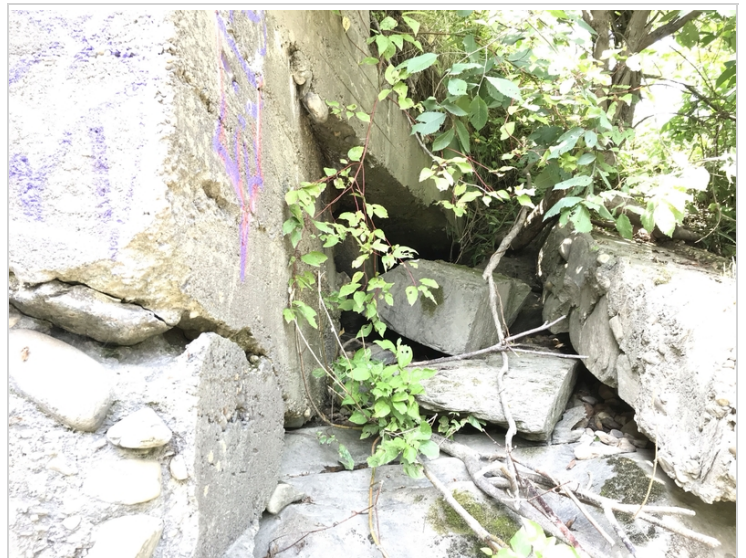
Downstream stream side of abutment 2
