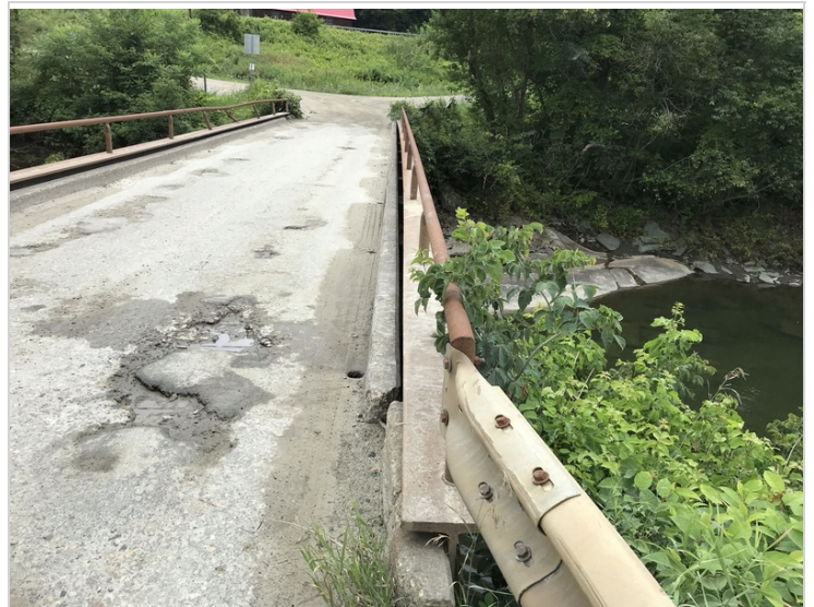
Downstream beam & rail from abutment 1
