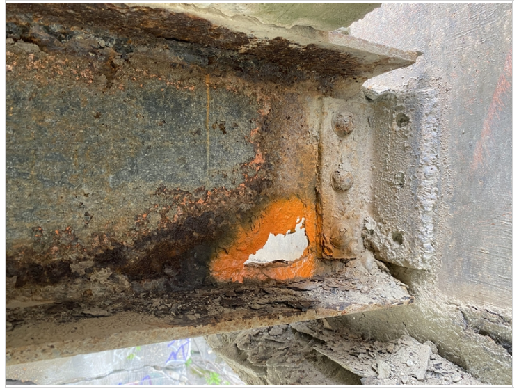
Floorbeam #7 on Downstream Side
