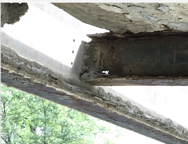
Downstream end of floor beam 7
