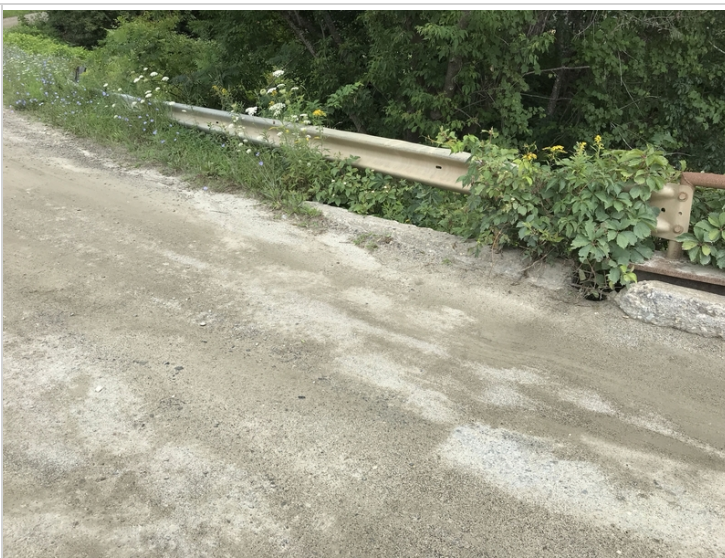
Downstream approach rail to abutment 2
