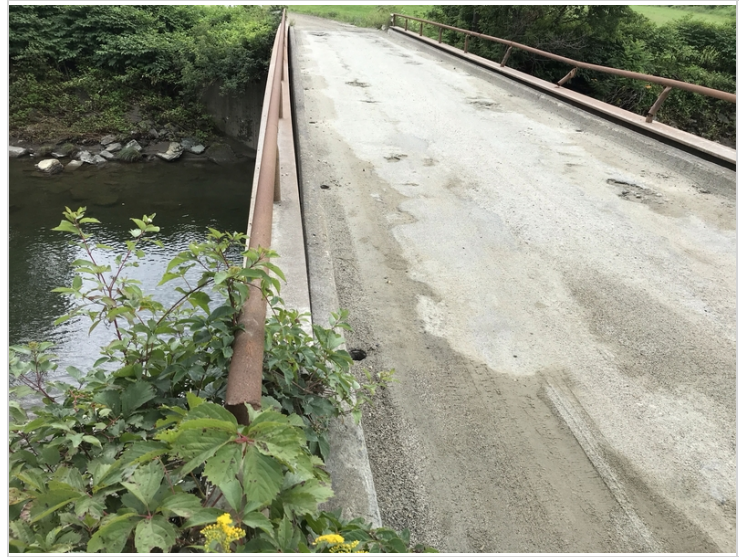
Downstream beam & rail from abutment 2
