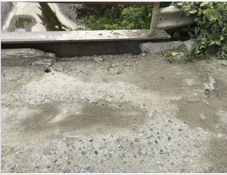
Upstream curb at abutment 2
