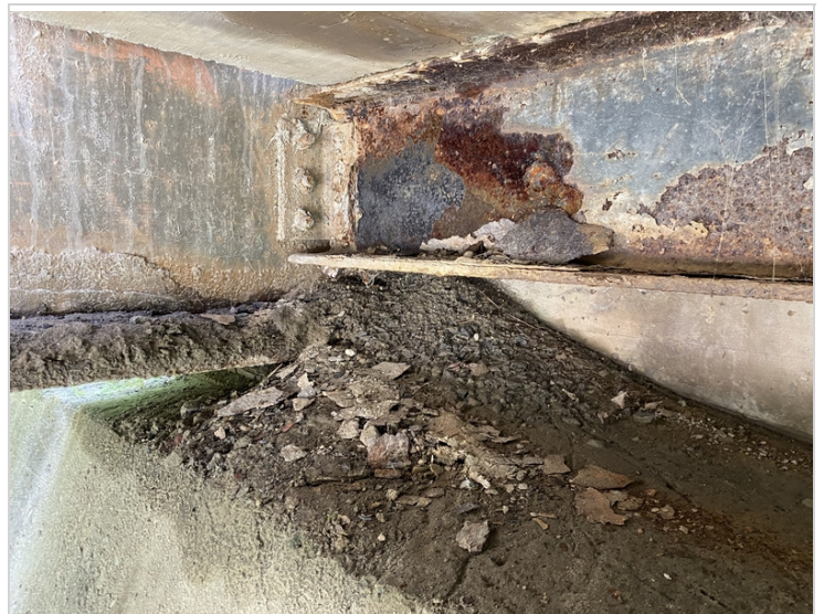
Floorbeam #0 on Downstream Side
