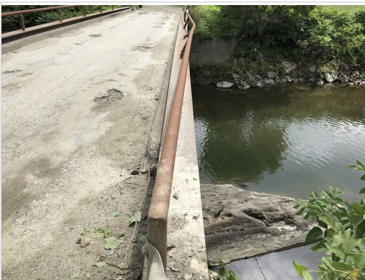
Upstream beam & rail from abutment 2
