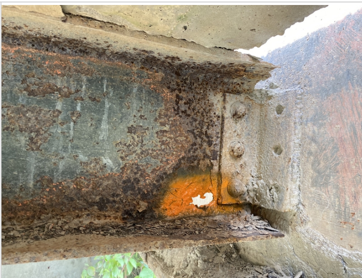
Floorbeam #8 on Downstream Side
