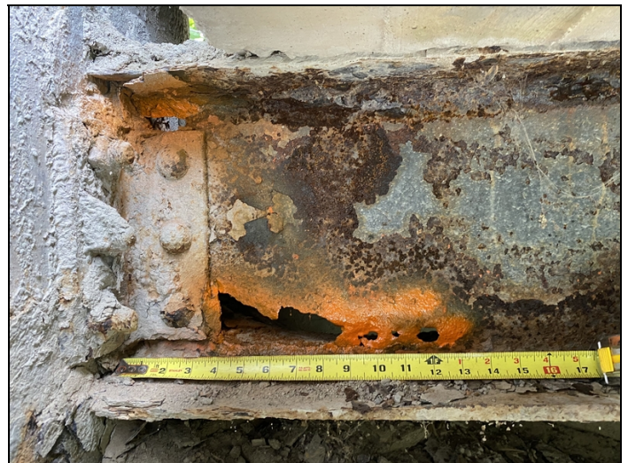
Floorbeam #9 on Upstream Side
