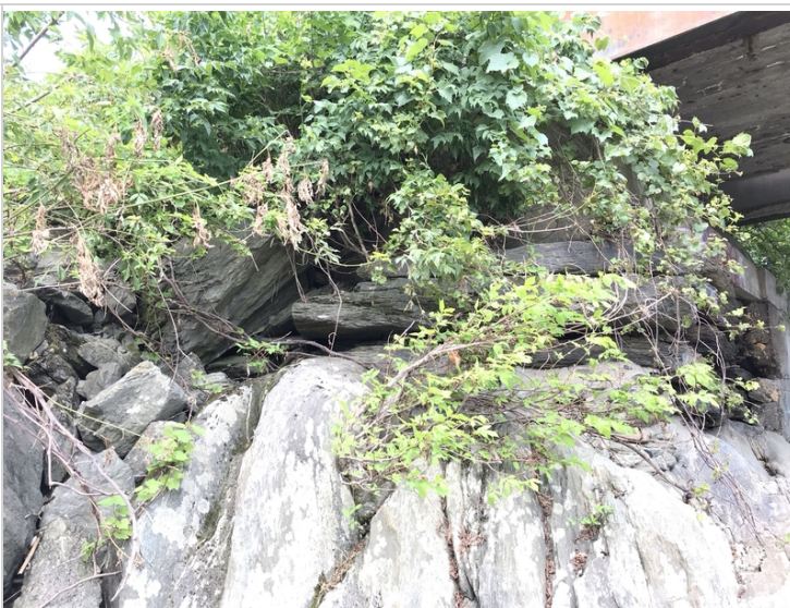
Upstream side of abutment 2
