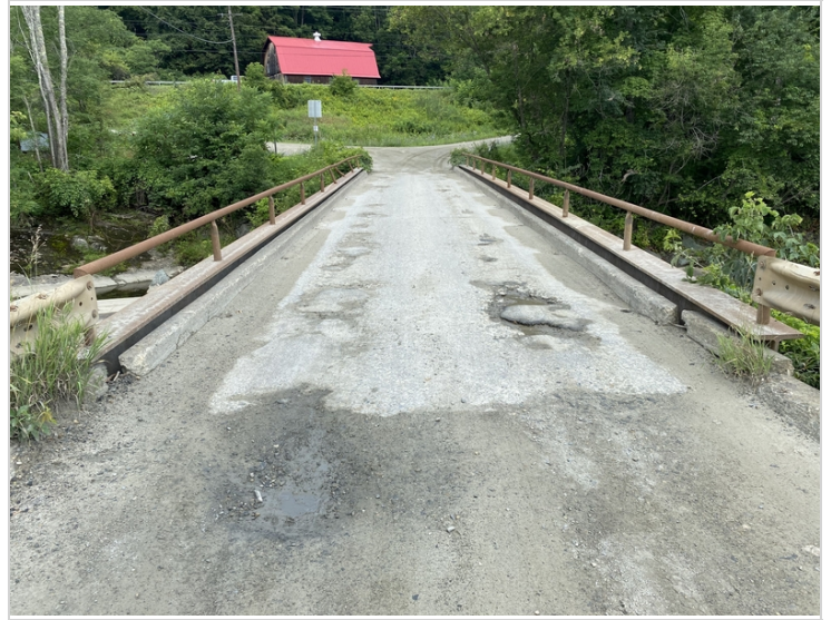
Top Surface of Deck from Abutment #1
