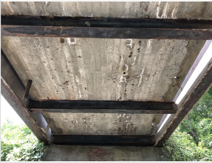
Soffit & superstructure facing abutment 2
