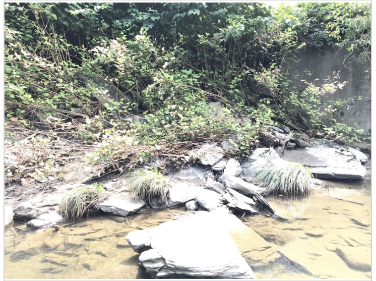
Downstream of abutment 1
