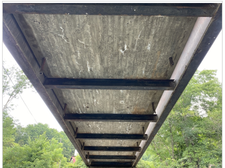
Deck from Abutment #1
