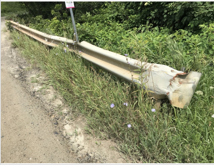
Downstream approach rail to abutment 1
