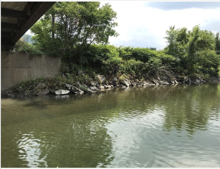
Upstream of Abutment 1
