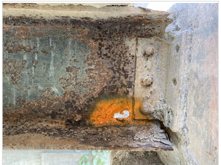
Floorbeam #8 on Downstream Side
