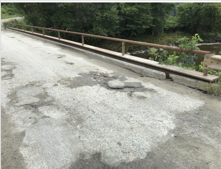
Downstream rail from abutment 1
