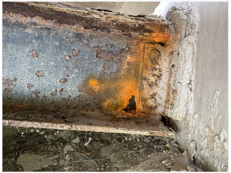
Floorbeam #9 on Downstream Side
