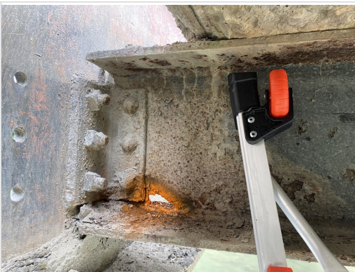
Floorbeam #6 on Downstream Side
