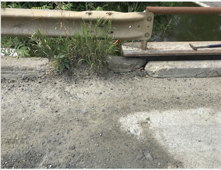
Upstream curb at abutment 1
