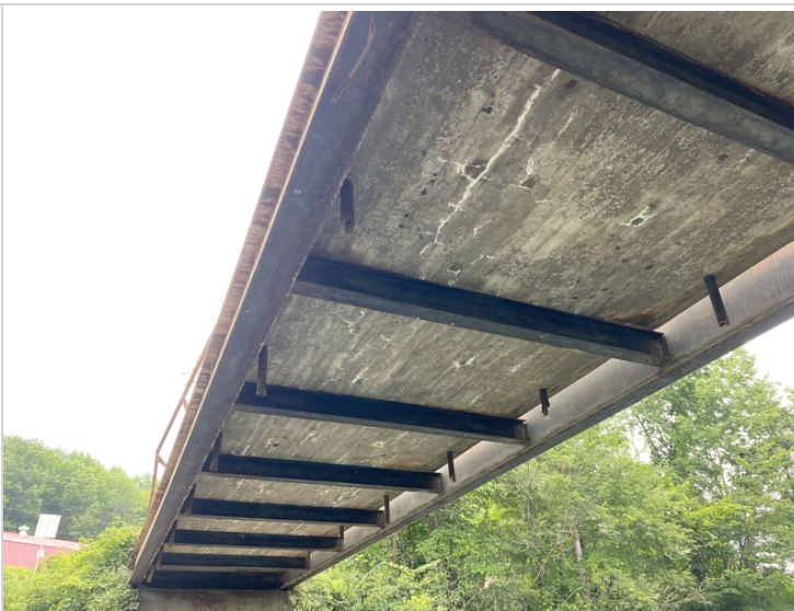
Superstructure from Abutment #1
