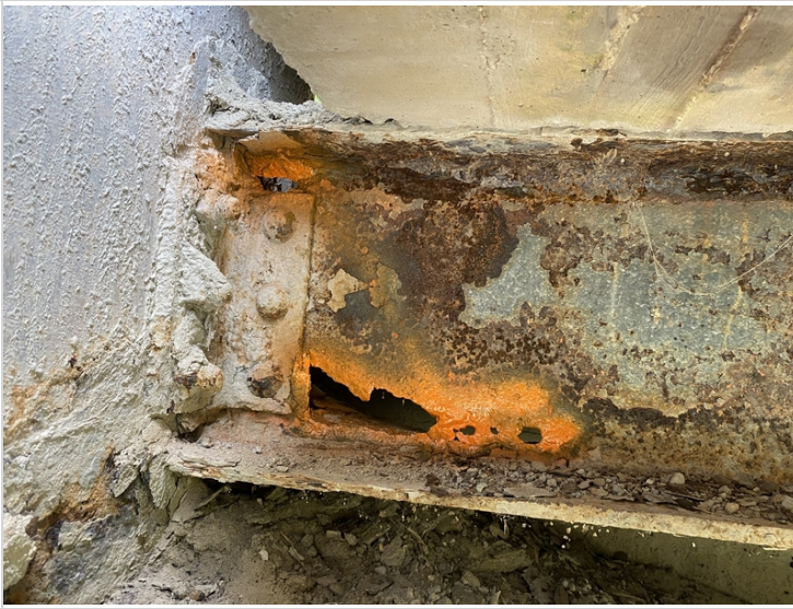
Floorbeam #9 on Upstream Side
