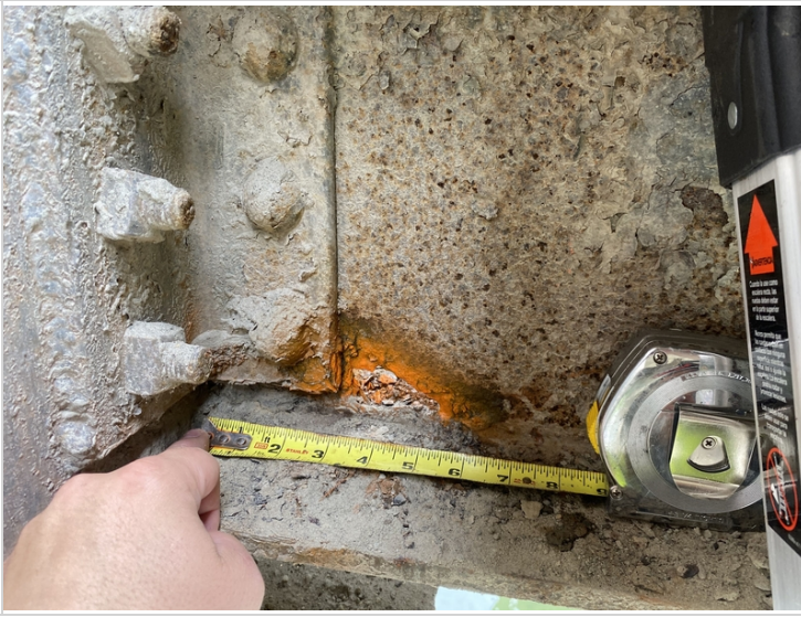
Floorbeam #6 on Downstream Side
