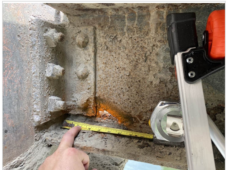
Floorbeam #6 on Downstream Side
